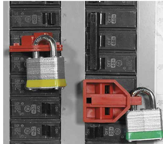
Application of Single Pole & Multi-Pole Breaker Lockouts
